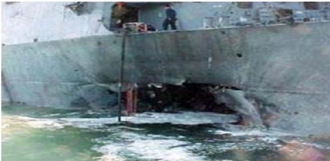
Figure 6.2.4: Close-Up of Hole in Hull of Cole
