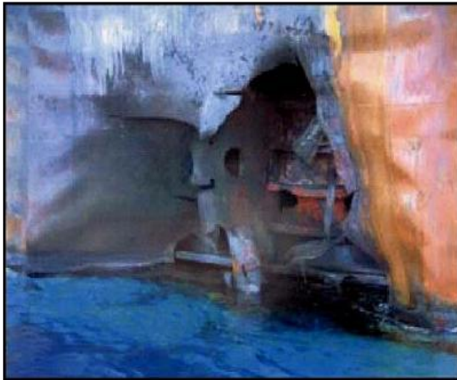
Figure 6.2.3-2: Close-Up of Hole in Hull of Limburg
